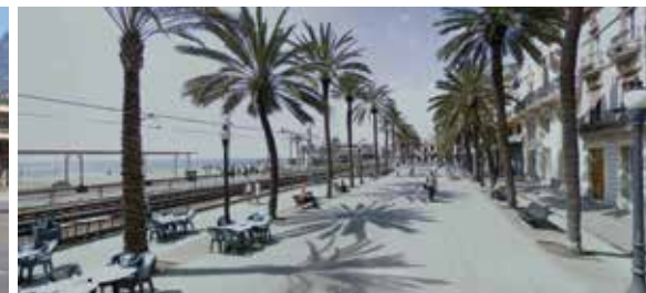
Transparency: visually connecting the waterfront, the rail and the city. Badalona, Spain
