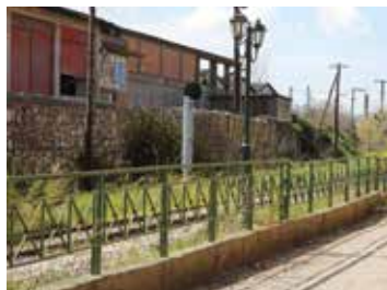
«yapi» respects existing corridor elements.
