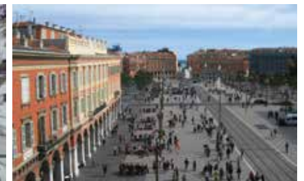
Rail stops become lively urban spaces. Historic city is extended. Nice, France
